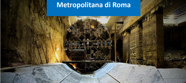
Rome Metro New Line C - T3 Section
